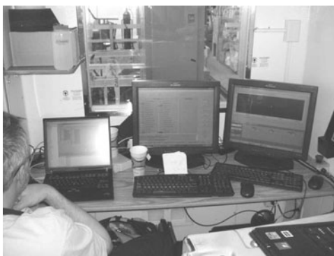
Fig. 10. Inside of control room.
