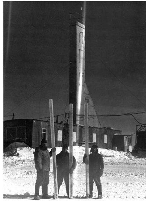
**Fig. 11.** Mean daily core production in SAE-32: three pieces of core, each with a length near 3 m.
