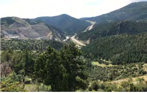
Looking East at I-70 as it descends Floyd Hill, crossing actively creeping slopes.
